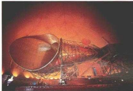
Radome-covered horn antenna at Andover, Maine, Earth Station.
